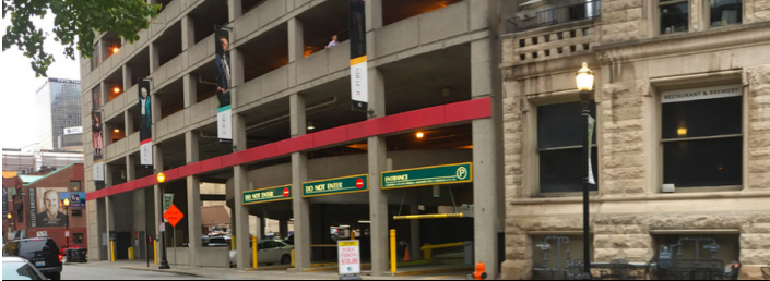
THIRD STREET PARKING ENTRANCE.
